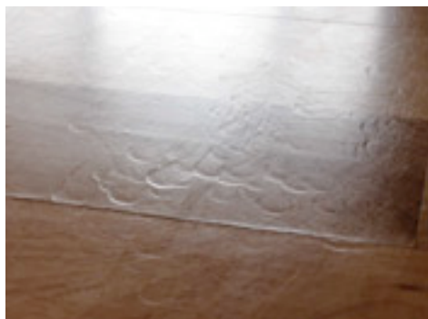
Dents, such as these from furniture legs, will not be hidden by recoating.
