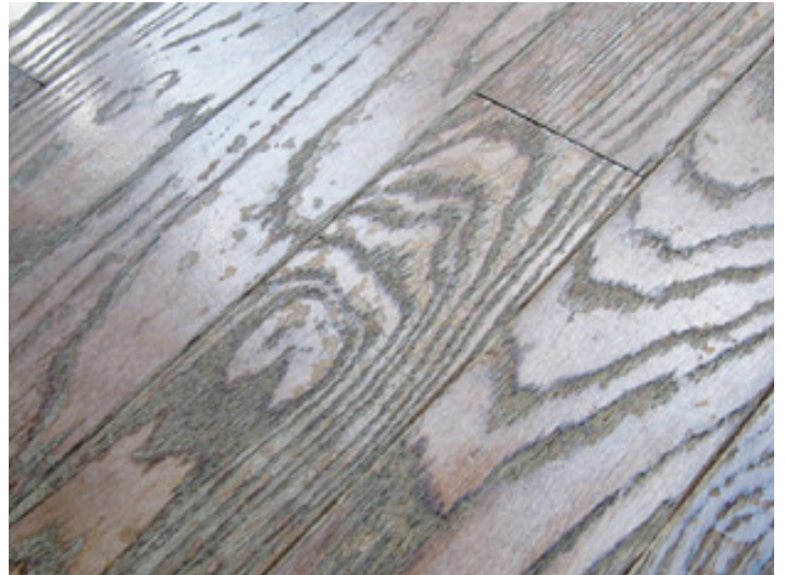
A prefinished solid wood floor damaged by repeated use of a steam mop cleaner.
